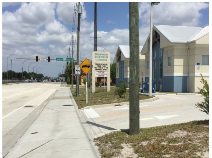
Looking North toward the fire station
